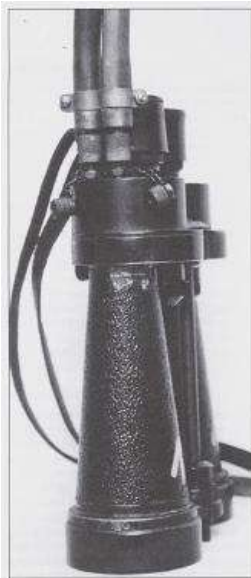
Fig. 3 Barr & Stroud CF41/AP1900A (WR/K017) in the process of desiccation. This binocular, serial no. 70119 was sold to the Admiralty in 1945. (Reid, note 4, op. cit., p. 172).
